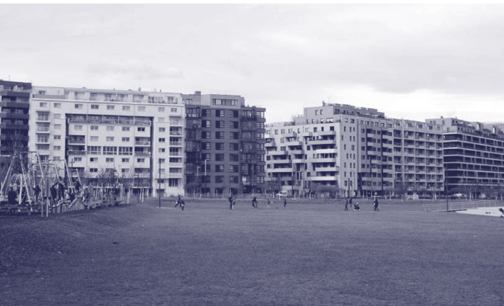
The new development at Vienna's railway station offers affordable housing and quality public space
